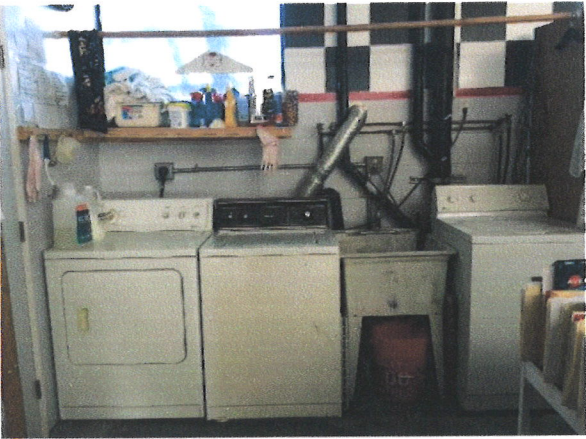
Washing Machines and Dryer
